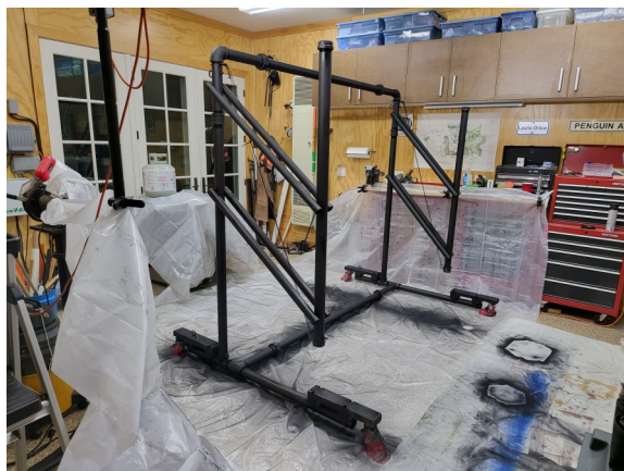
The video wall frame under construction in the Orlow workshop.
